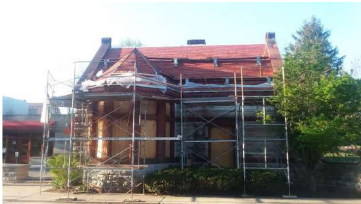
The Administration Building with its newly-tiled roof.
