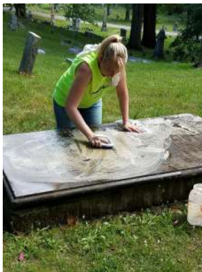
Misti works on the David Ziegler monument removing biological growth and staining. Below, the remarkable transformation that allows for the reading of the ledger.
