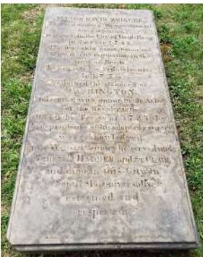
Misti works on the David Ziegler monument removing biological growth and staining. Below, the remarkable transformation that allows for the reading of the ledger.
